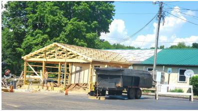
The new restroom project is coming along with footers poured and the first posts installed. Framing the addition is done as well as some underground plumbing and some inspections were accomplished. Tie ins of the addition roof to the existing roof were also successfully made.
